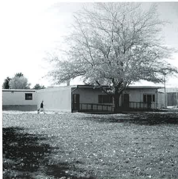
T901-T906 Temporary modular Classrooms South of the Art Complex
