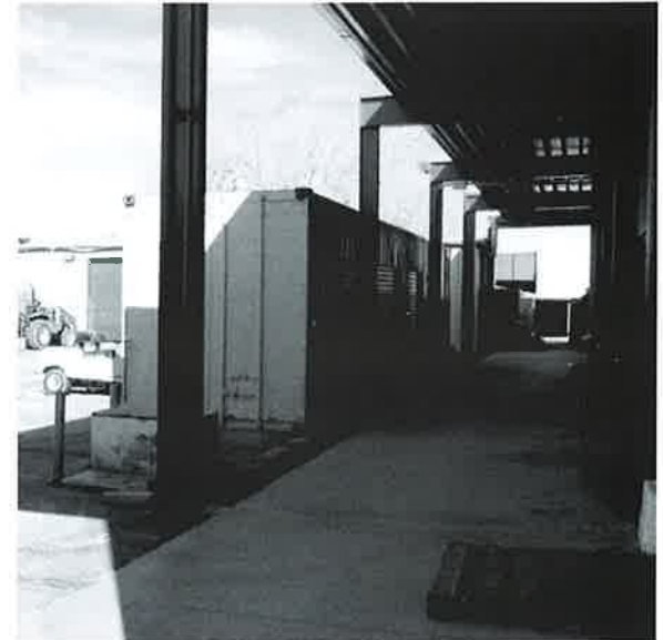
Electronic and Welding Shops Storage Containers Behind Existing F2 Building
