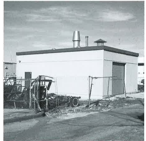
Existing Paint Booth South of Maintenance and Operations Complex
