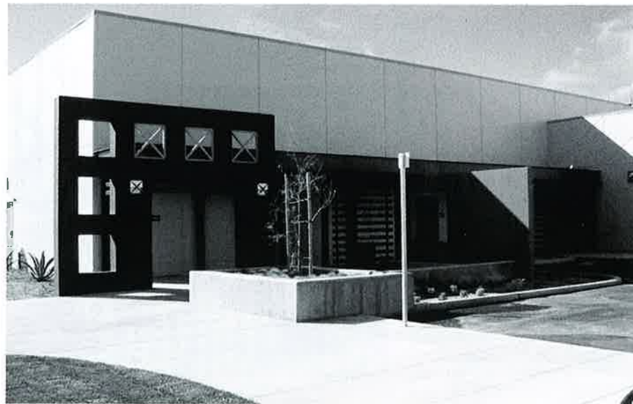
Antelope Valley College Advance Technology Building 2003. This project was identified in the previous 1992 Facilities Master Plan.
