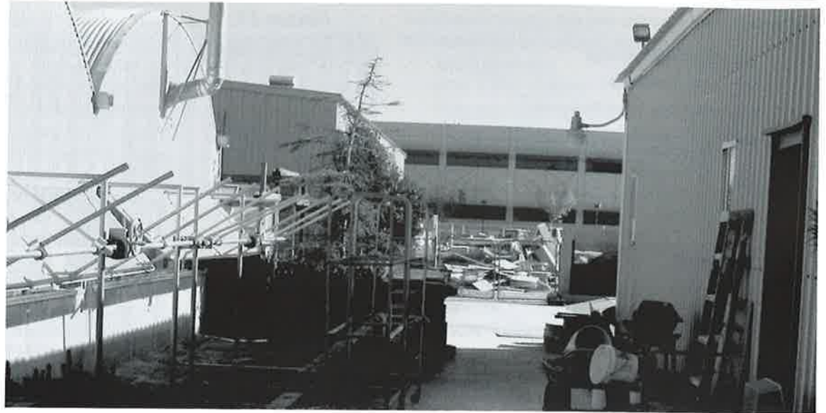
Existing greenhouses and storage building
