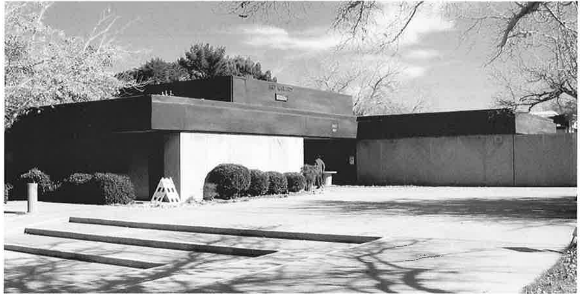
Exterior of C-I Ceramics Building Located in the Fine Arts Complex
