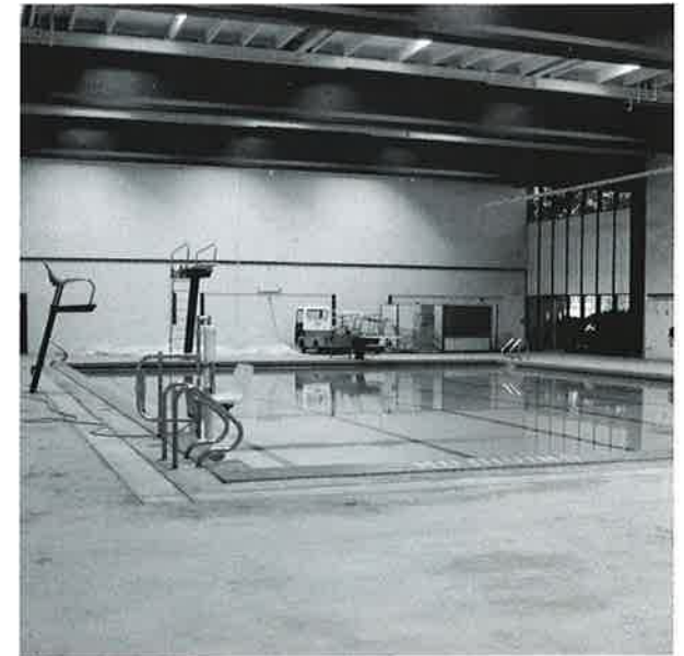
Existing Pool Interior Pool Facility
