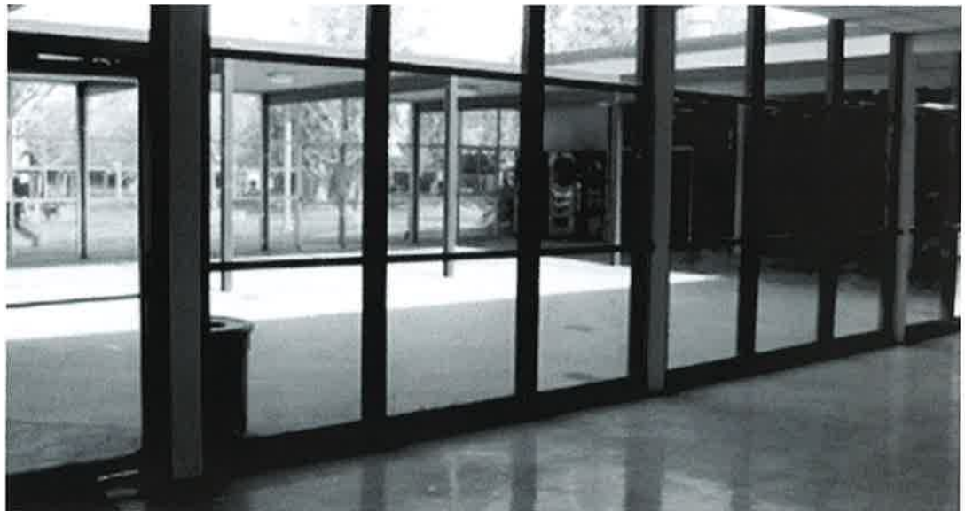
Student Center courtyard to be enclosed to provide additional space to the existing book store and a more fluid connection between interior spaces
