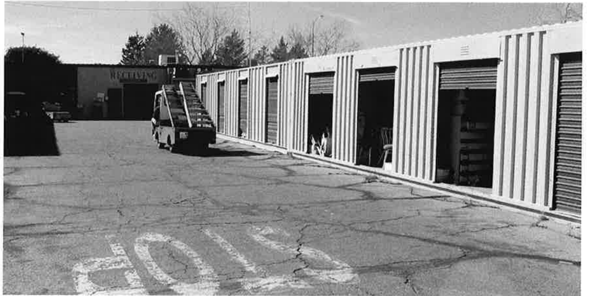
Maintenance and Operations Storage Containers
