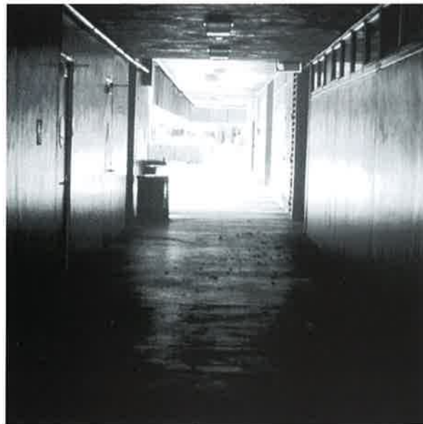
Existing Humanities Exterior Corridor
