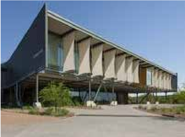
Vertical shade structures at north facing glazing protect from western sun while providing interest to elevation.
