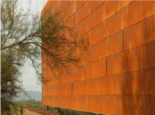
Weathered steel with protective patina provides durable finish.
