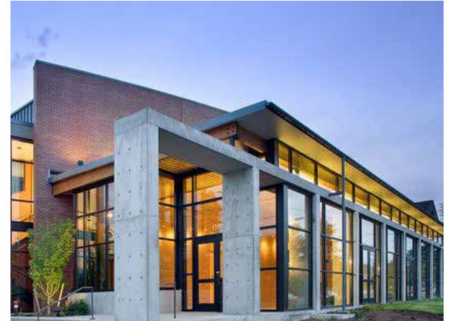
Structural system expressed in facade
