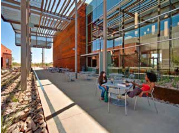
Steel trellis provides shading of south facing glazing.
