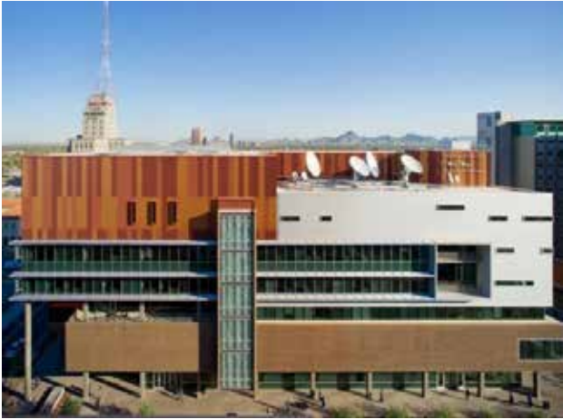
Massing as well as varied patterns, materials expressed in an orthogonal manner.
