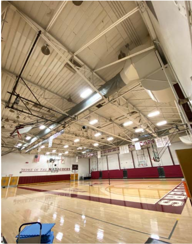
EXISTING BUILDING JANUARY 21, 2020
