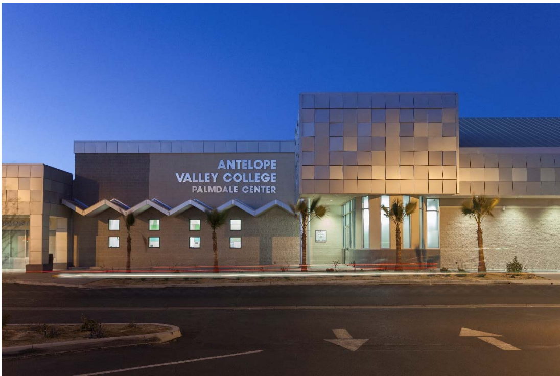
COMPLETED BUILDING OCTOBER 26, 2017
