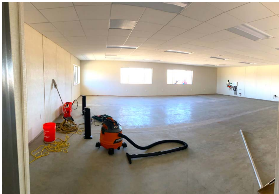
FOX FIELD; CLASSROOM PROGRESS JANUARY 14, 2020
