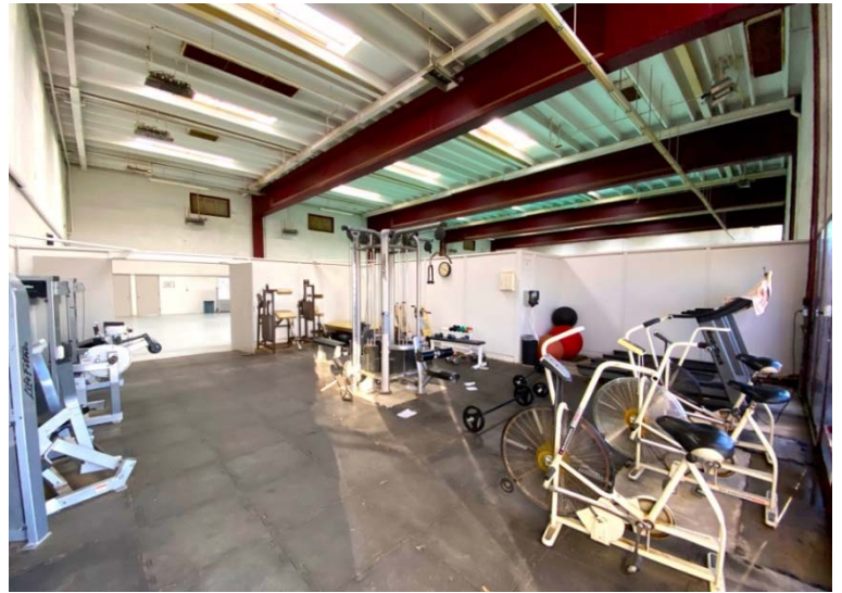
EXISTING BUILDING JANUARY 21, 2020
