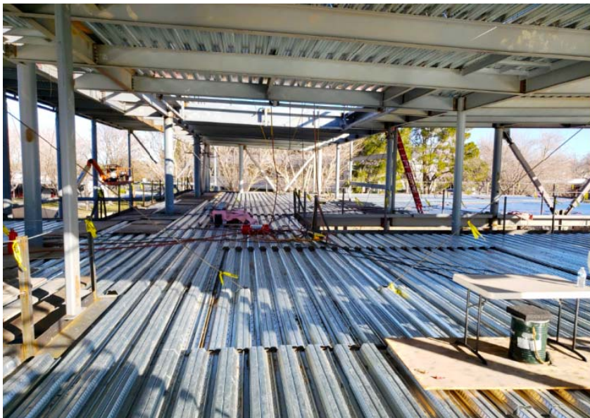
SAGE HALL PROGRESS January 22, 2020
