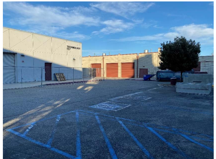
DISCOVERY LAB EXISTING SITE JANUARY 21, 2020
