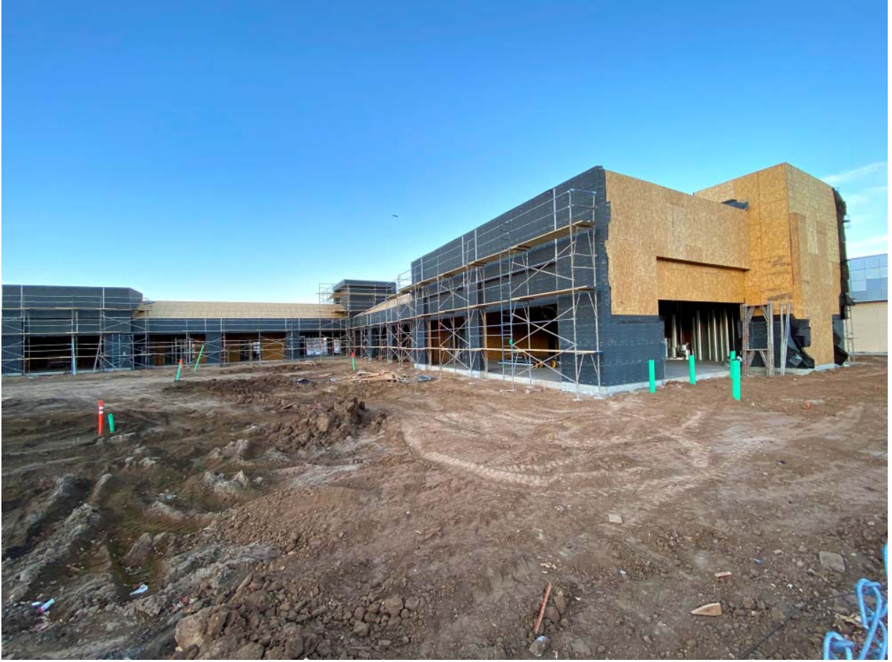
EXISTING SITE / PROGRESS JANUARY 21, 2020
