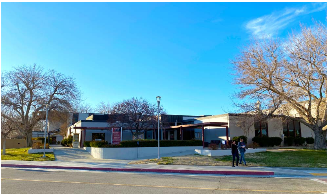
EXISTING SITE; FUTURE CEDAR HALL JANUARY 21, 2020
