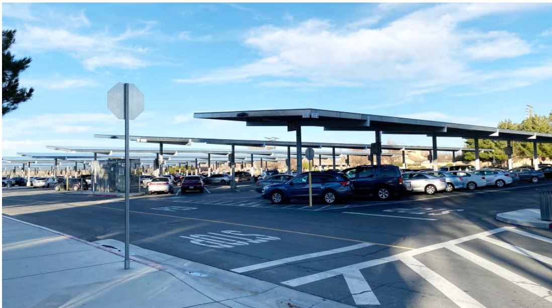
EXISTING PHOTOVOLTAIC ARRAYS TO BE RELOCATED JANUARY 21, 2020
