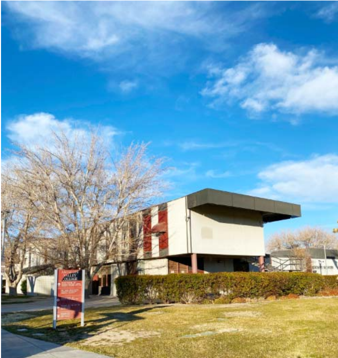
EXISTING SITE; FUTURE CEDAR HALL JANUARY 21, 2020
