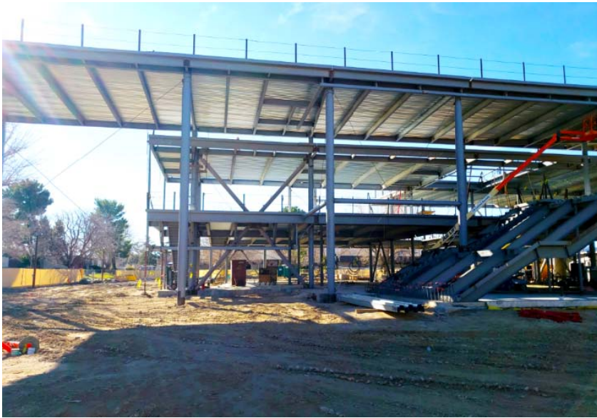
SAGE HALL PROGRESS January 22, 2020
