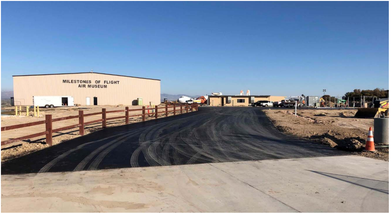
FOX FIELD IMPROVEMENTS; PROGRESS JANUARY 29, 2020
